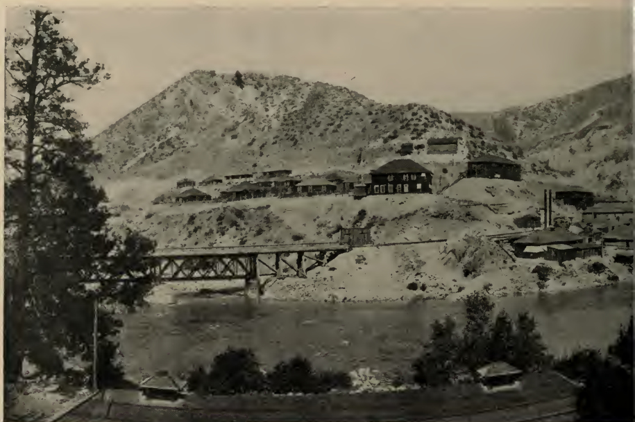
LOCATION OF ARROW ROCK DAM. 351 FEET I
