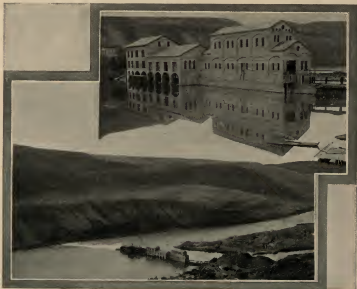
Swan Falls Dam and Power Plant on Snake River Generating Light and Power for Boise
