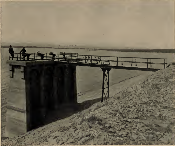
Outlet Gates at Deer Flat Reservoir, Boise Reclamation Project
