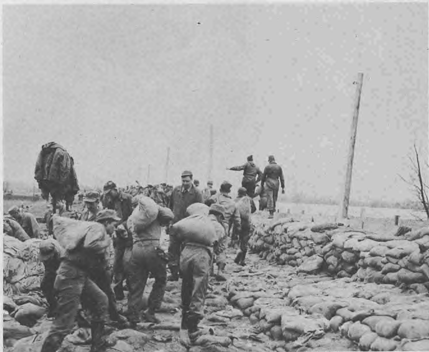
4. Council Bluffs No. 14 St. levee, sandbag operations on levee by 201st Brigade from Camp McCoy, Wis.
