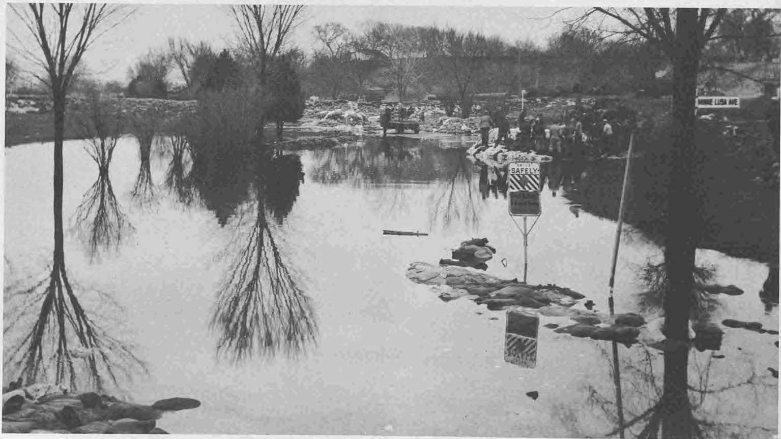
44. Omaha. Backwater—Pershing and Minne Lusa, sandbagging.
