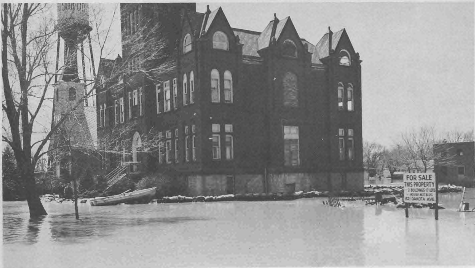
39. So. Sioux City, Neb. Church located on Dakota Ave. next to City Hall. Notice sand bag protection.
