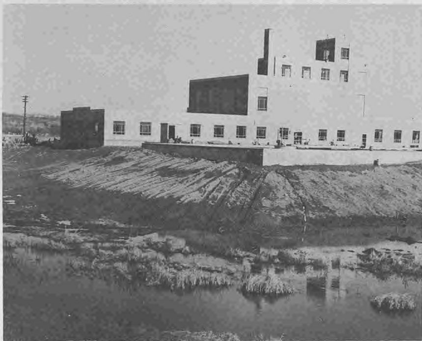
6. Water purification plant in Council Bluffs. Note earth piled and bags in front.
