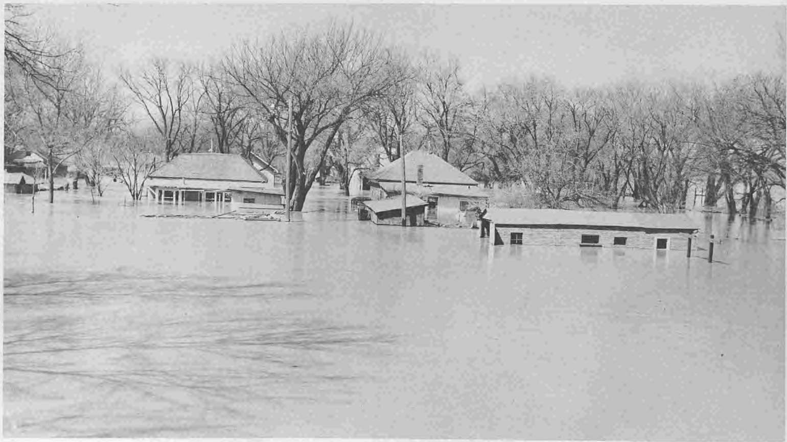
40. So. Sioux City, Neb. Buildings at foot of bridge leading to Sioux City proper, completely inundated.
