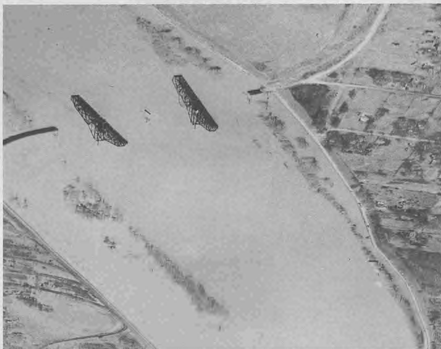
5. Council Bluffs Dike which bore the brunt of the water's fury. A few miles further upstream the river fanned out to a fantastic width of twelve miles.
