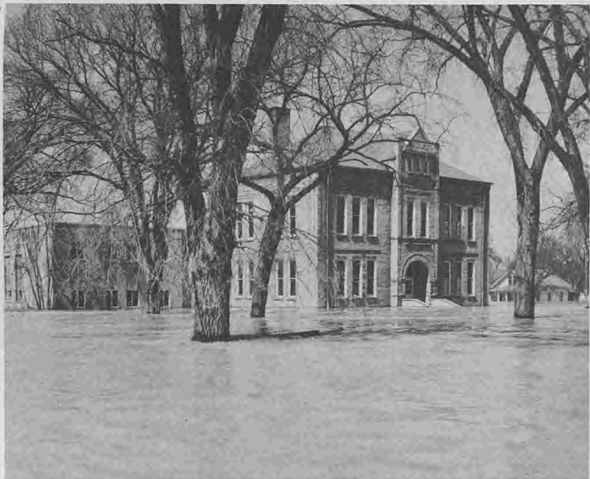
48. So. Sioux City. Public school building partially under water. No school today.
