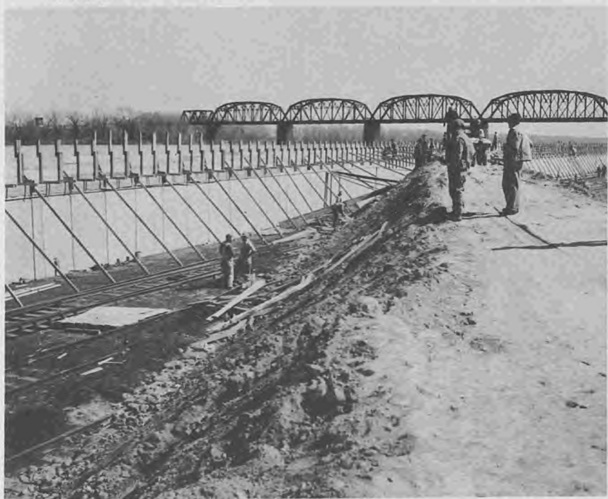
7. Omaha. Looking south on new back levees being built at Jones St. Pumping Station.
