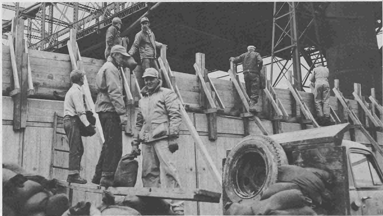
16. Added height and strength was given to the Omaha floodwall by the Corps of Engineers with the construction of flashboarding backed with sandbagging.
