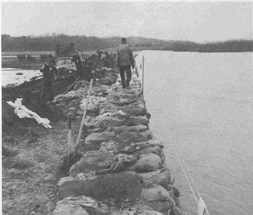
50. Ft. Leavenworth, Kansas. Building levee at Sherman Field. Workers on levee.
