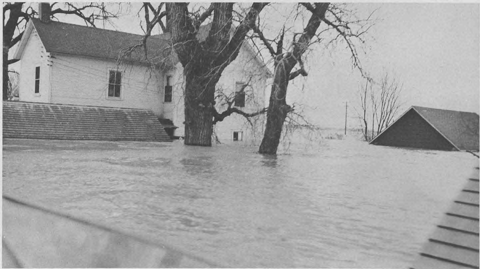
14. Near Florence, farm house inundated—stage approximately 29.5.
