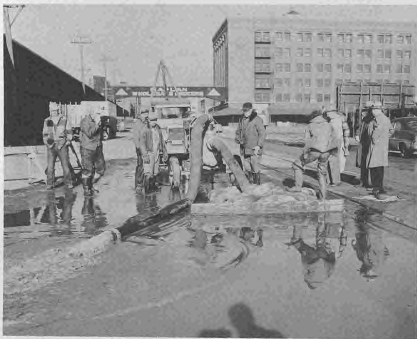
46. Sioux City, Iowa. City Engineer and George Neal, President of Iowa Public Service Co., supervising installation of pump which is removing water from sanitary sewer to street level.
