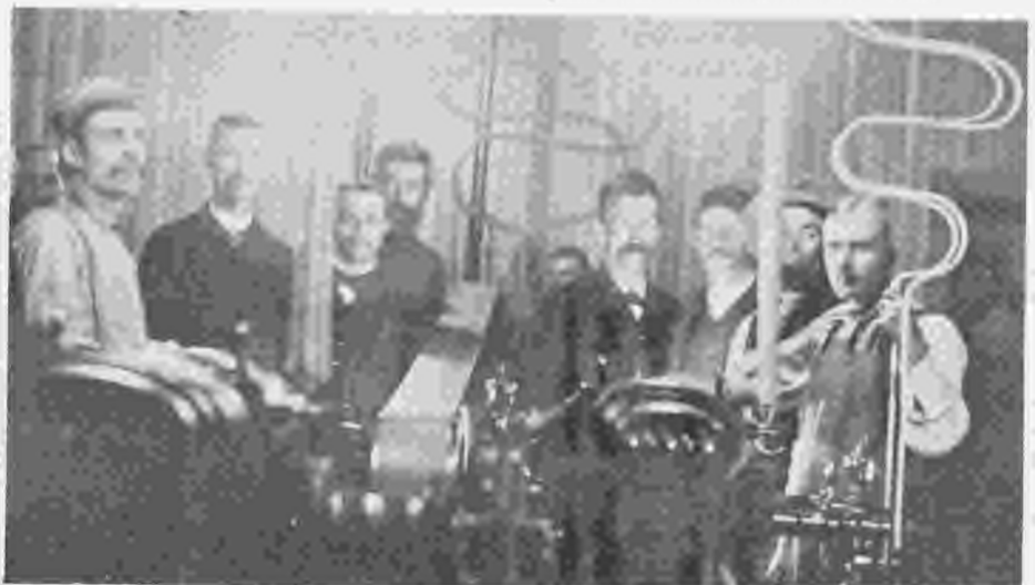
GREAT BEND'S FIRST ELECTRIC PLANT—1885
