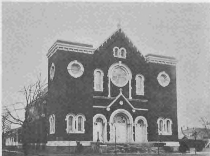
St. Rose of Lima Catholic Church; new building constructed in 1915.
