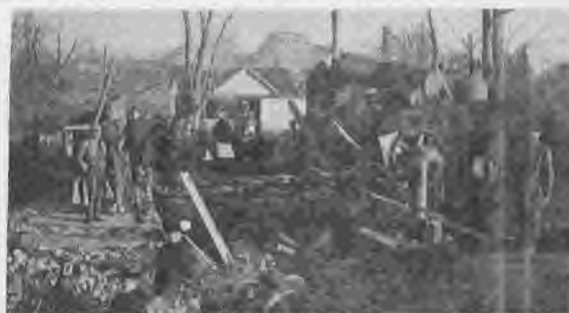
Great Bend Water Company showing wrecked pumping station and water tower.
