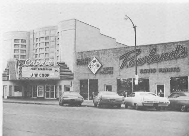
The south side of the Square.
