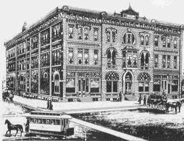
THE MORRISON, AS DESIGNED & BUILT BY MORRISON BROS. GENERAL CONTRACTORS & BUILDERS N. E. CORNER LA FAYETTE PARK, GREAT BEND, KANSAS
