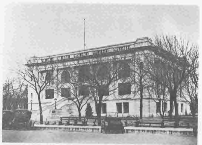
The courthouse you see in 1972 was constructed in 1918. This 1920 view from the west shows the long steps which were taken off in about 1948.
