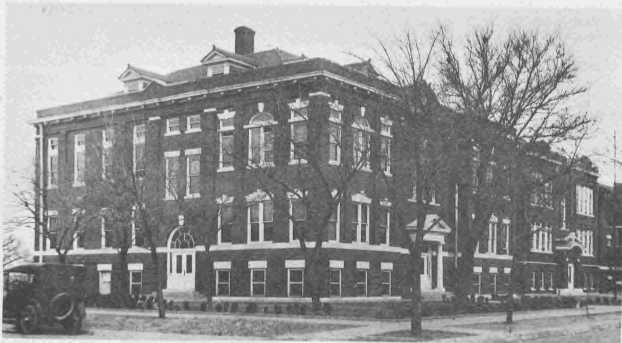
The high school and Central School building, in the 2100 block of Forest, were razed in 1970 to allow construction of the new public library.
