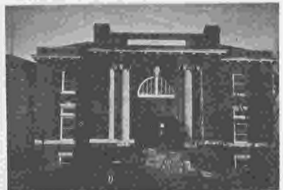
Under construction in 1908.
