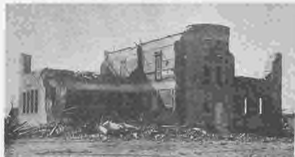
Roosevelt School wrecked by the 1915 Tornado.
