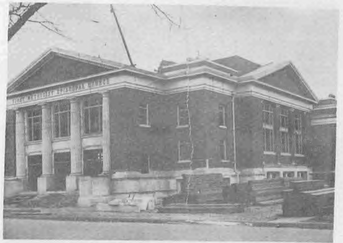
The First Methodist Church in construction in 1920.
