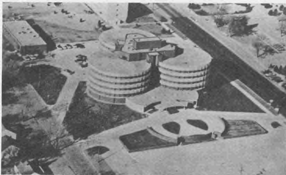
Aerial view of the Central Kansas Medical Center showing the circular cloverleaf design.
