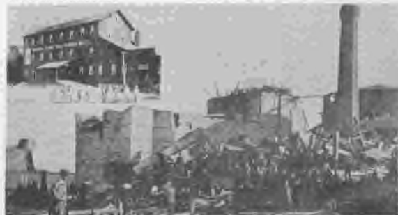
Walnut Creek Flour Mill before and after the cyclone.
