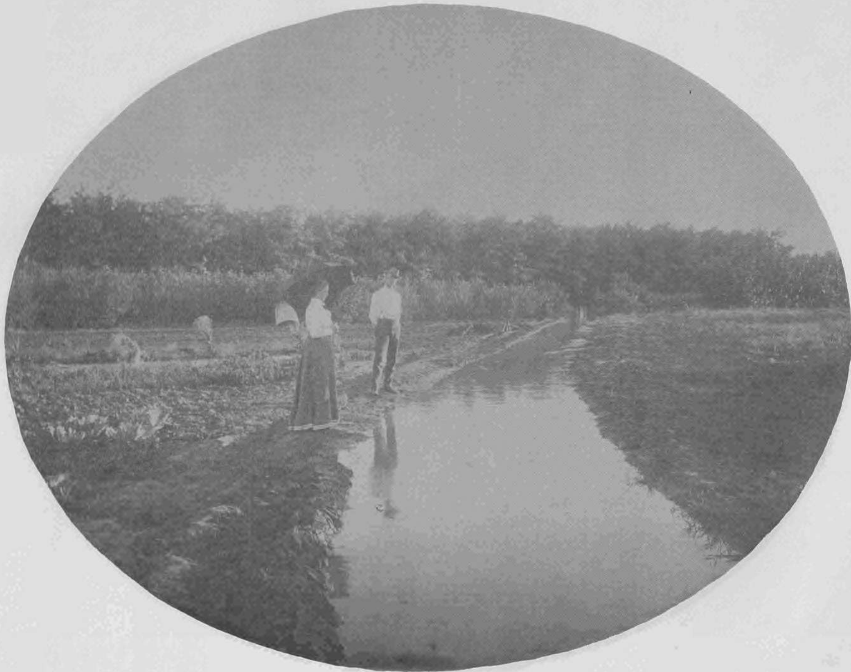
Col. Perry's irrigation ditch near Englewood, Kansas, in 1896. Col. Perry has extensive Alfalfa fields as well as the orchard seen here.
