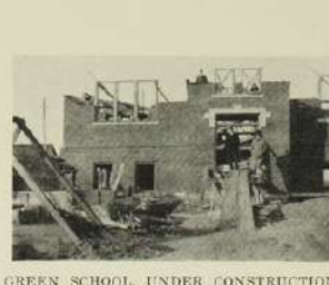
GREEN SCHOOL, UNDER CONSTRUCTION. Built by Samsman Bros., GREEN, KANSAS.
