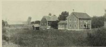
BUILDINGS ON FARM OF JOHN KOERFER, GREEN, KANSAS.
