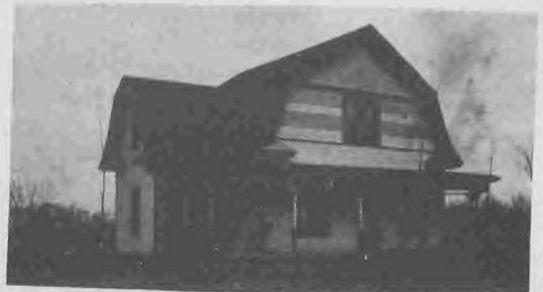
The Mauck Brothers built this house for James Jacobs in 1908. It was salvaged by the U. S. Government. Occupants known were: James Jacobs, John Shobe, Verna Cochran and Mrs. Josephine Baker and grandson Melvin Darbyshire.
