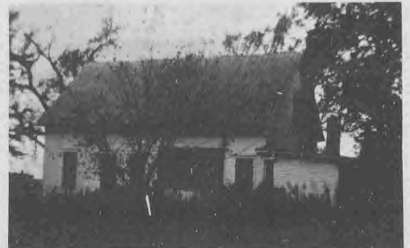
Northwest of Strawn-Wm. Newkirk built this house in 1880. It still stands. Occupants known were: Jess Baxter, Peter G. Metzler, Kenneth Hamman, Clarence Baxter, Silas Laws, Walter Laws, Carl Williamson, Hugh Dalrymple and Donald Williamson.
