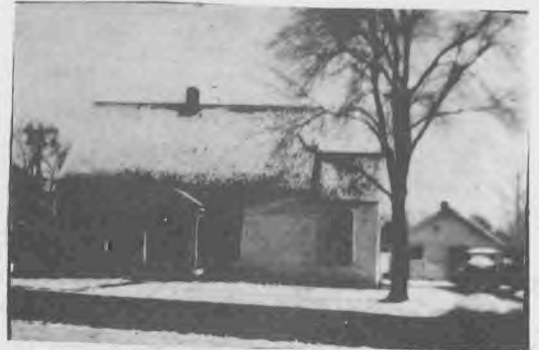
Dudley Doolittle built this house for Conrad Hamman in 1911 for rental. It was remodeled by Howard Claycamp in 1947. It was purchased by Mr. Dunn and moved to Neosho Rapids, Kansas. Occupants known were: W. E. Hughes, S. T. Anderson, Joe Mayer, Charles Hamman, Alfred Farmer and Howard Claycamp, 1932-63.
