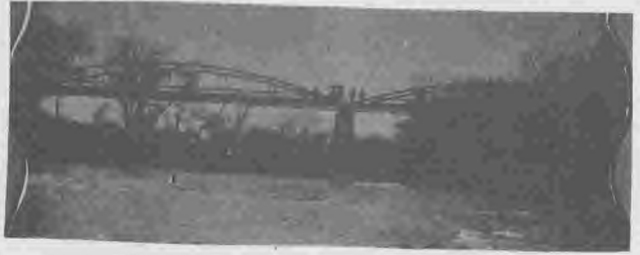
First Neosho River bridge.
