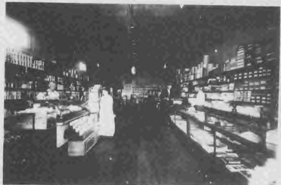
Inside the Hoover Store-Lillie Means, Silas Hoover and Harry McCormick behind the counter.
