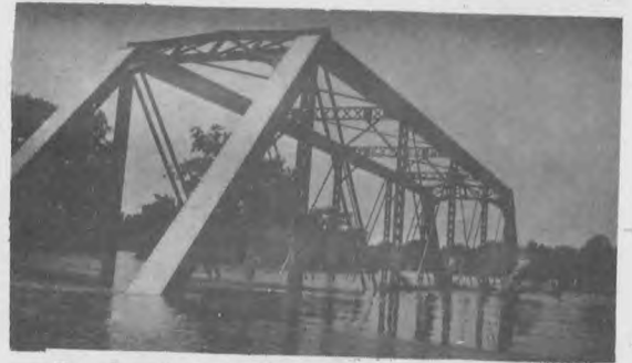
Eagle Creek MK&T (Katy) bridge.
