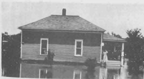
Pratt Williamson moved this house from Gas City, Kansas. It was cut in two parts and moved on the Katy railroad. It was purchased by Wm. Pickett. Occupants known were: Lee Baysinger, W. C. Pennybaker, Elsie Danner, Edgar Williamson and Frances Crooks.
