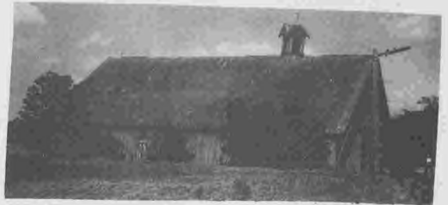
Jacobs barn was built in 1886 of North Carolina pine. The stales were walnut and the barn was put together with wooden pegs. It was salvaged for lumber in the 1950's and in very good condition.
