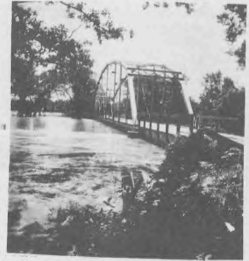
Neosho River bridge.
