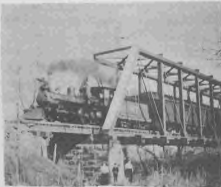
Eagle Creek MK&T (Katy) bridge.
