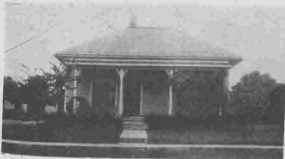
Charles Hamman built this house in 1914. It was moved to New Strawn, Kansas. Occupants known were: Chas. Hamman, Earl Pennybaker, Dr. Zimri Houser, A. J. Bauer, Harry Duckett, Roy Johnson and Clarence Baxter.
