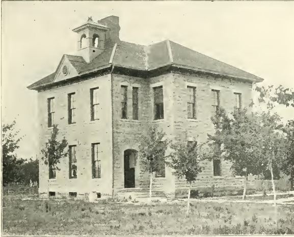
EAST WARD SCHOOL, WINFIELD
