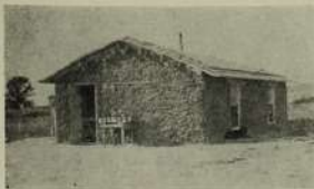
PIONEER SOD HOUSE, Former Residence of Roy Chilson, OBERLIN, KANSAS.
