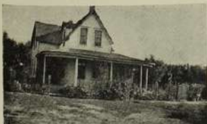
RESIDENCE OF GERHARD BOOR, SELDEN, KANSAS.
