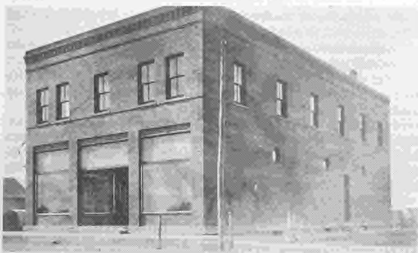
The Erickson building when it was a two-story building.
