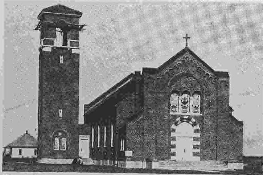
Church photo when construction was still underway on the bell tower.
