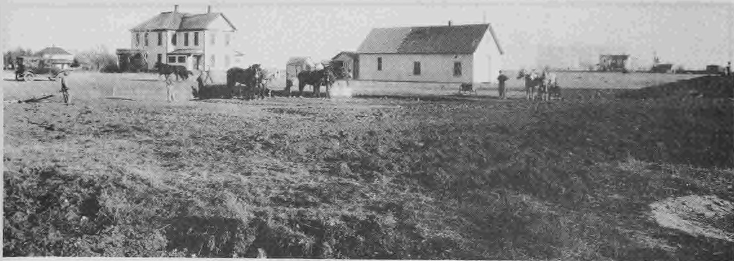
Groundbreaking for present St. Bernard's Church.
