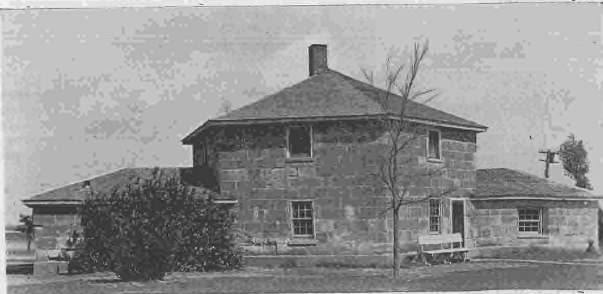
The Block House, an unusually well preserved structure, was used as a headquarters building at Fort Hays. Built in 1867, it is hexagonal in shape and evidently had lookouts on the second story for there are loopholes in the masonry. It was used for a golf club house for a time and now houses the Old Fort Museum.
