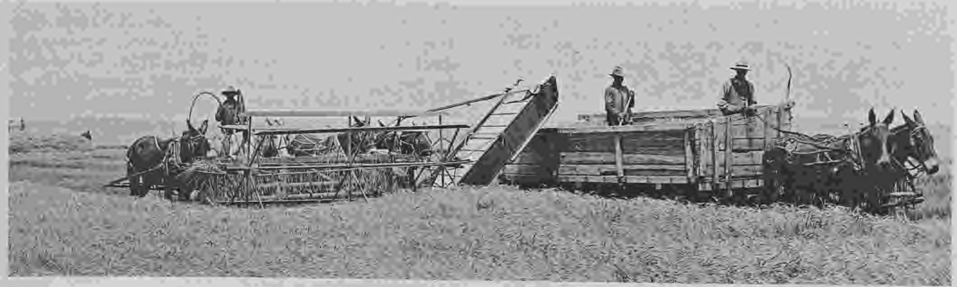
The header-barge, a popular early-day method of harvesting wheat in Ellis County.
