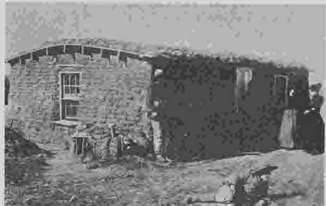
An early-day sod house typical of the first dwellings of many of the German-Russian settlers.
