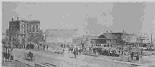
Devastation of the fire of 1895 in which eighty-seven business buildings burned.
