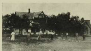
RESIDENCE OF CHAS HEITSCHMIDT, LORRAINE, KANSAS.
