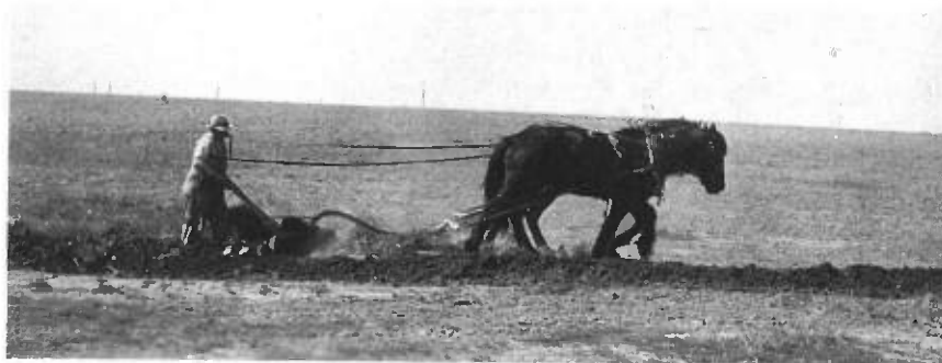
Breaking out sod west of Dodge City.
