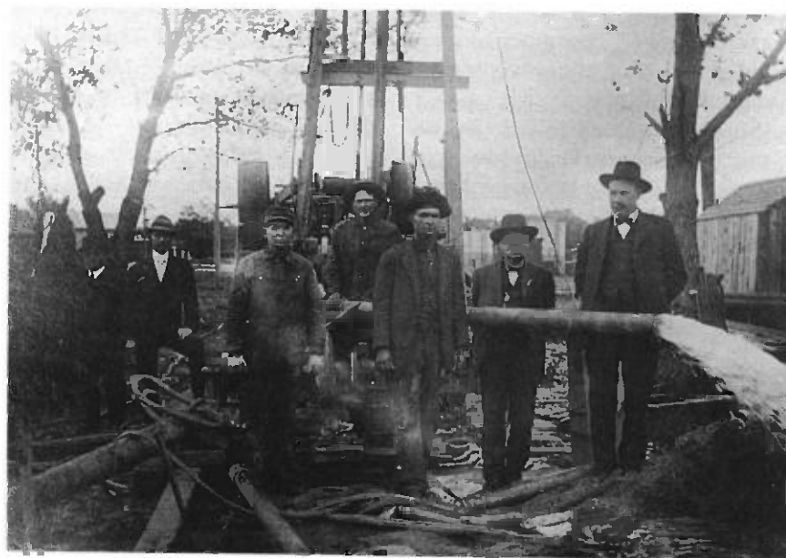
Dodge City's first deep water well. The official analysis was 99.+% pure. John Miller is pictured with his hand on his knee. Bert Johnson is in the center behind the pipe. Others behind the pipe are Sid Reynolds and A. Gluck, the mayor. In front of the pipe are Holly Forsythe and Oscar Johnson. The drilling rig belonged to Oscar Johnson.
