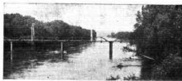
RIVER AND ELECTRIC RAILWAY BRIDGE, JUNCTION CITY, KANSAS.
