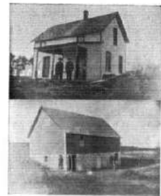
RESIDENCE AND BARN OF FRED SCHWITZER.
