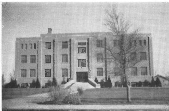
The present County Court House of Grant County, built in 1930
