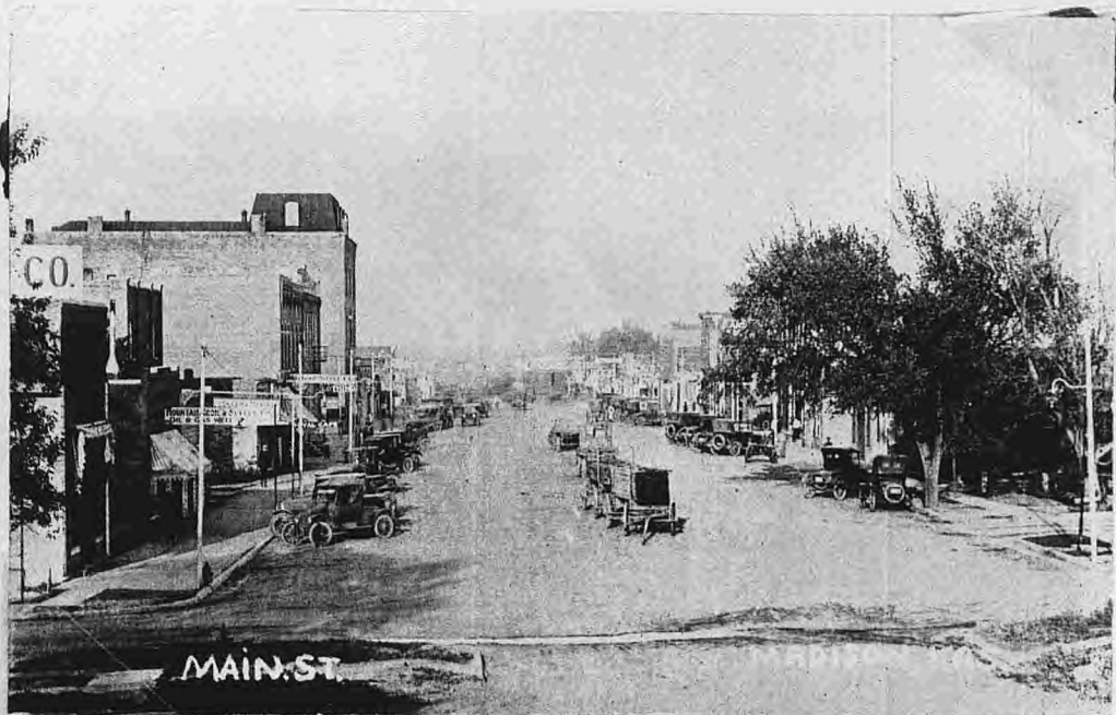
The loads of lumber sitting in the middle of the street were there in preparation for laying sidewalks.
