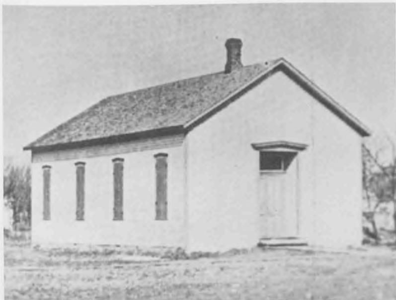
School-church facility erected in 1878.
