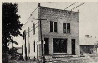
AMERICAN TELEPHONE COMPANY, HOLTON, KANSAS
