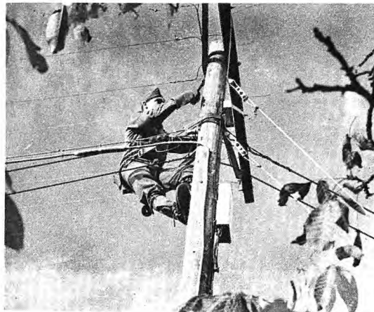
Pole Climber--Corporal Gerald Reser, of Oskaloosa, Kansas demonstrates proper form in working atop a pole used in wire communications. Corporal Reser is an instructor in pole line foreman work at the Western Signal Corps School, Davis, California, part of the Western Signal Corps Training Center at Camp Kohler, California.
