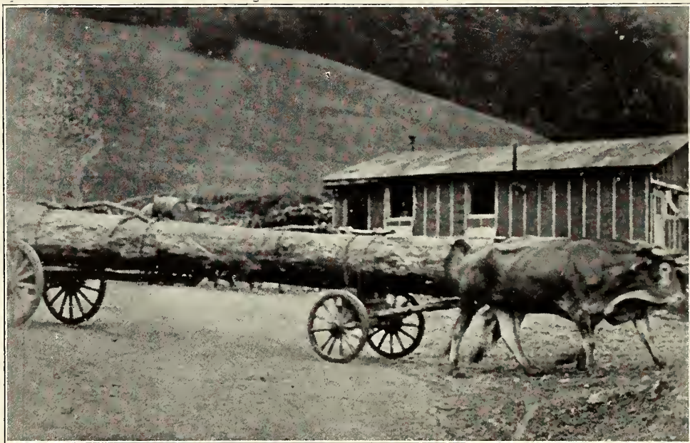
Logs arriving by ox-cart from adjoining woods, Co. C, 110th Engineers, Holsplatz, France, August 10, 1918
