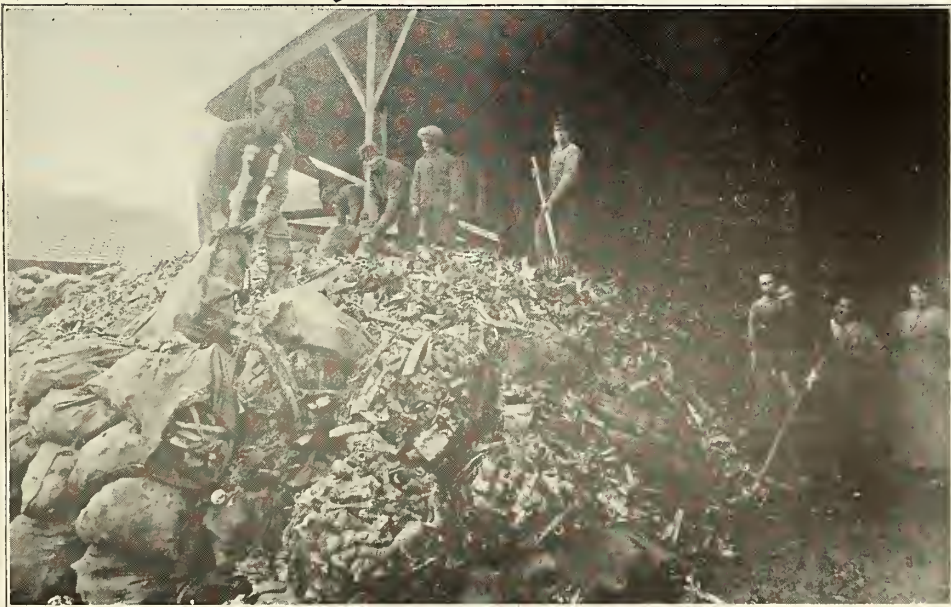
Piling 'em up in France
