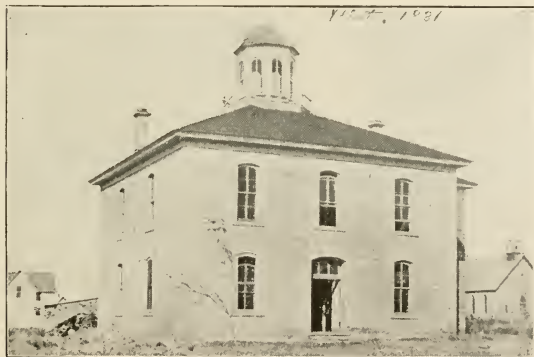
BUILDING THE COURT HOUSE.
