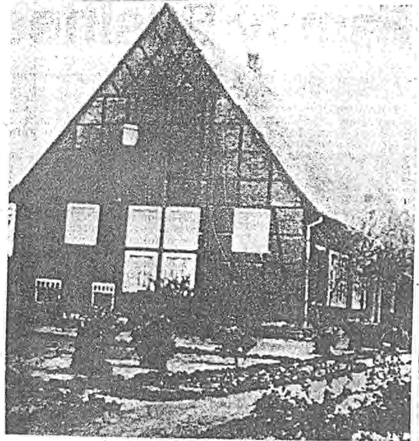
THIS RED BRICK, TWO-STORY HOUSE at Enniger, West Germany, is 120 years old. It was built in 1864 by Bernhard Heinrich Schockmann, great-grandfather of Mrs. Robert Smith, Ponca City. He came to the U.S. in 1882, settling in Coffeyville, Kan. Mrs. Smith, her husband and a cousin visited the German community last summer. Photo was taken in about 1930.
