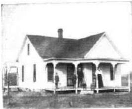
Residence of Wm. CRAPSON
