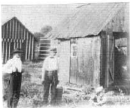
Pumping Station of JAMES T. SMITH
