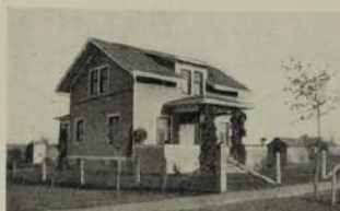
RESIDENCE OF E. E. JETHR, Owner and Publisher of the Lenora News, LENORA, KAN.
