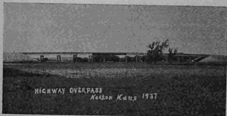
The Railroad Overpass, Norton
