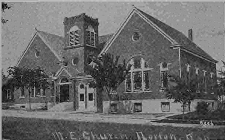
METHODIST CHURCH, North State Street, established in March, 1876. Above church erected 1905. Among charter members were David Close, Eli Dopps, Lizzie Dopps, D. M. Robinson and Mrs. D. M. Robinson. Rev. M. C. Brooks, Pastor, 1940--
