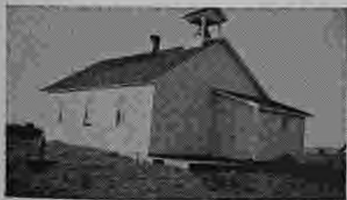
District Number 17 School. (Cracker Box Type)
