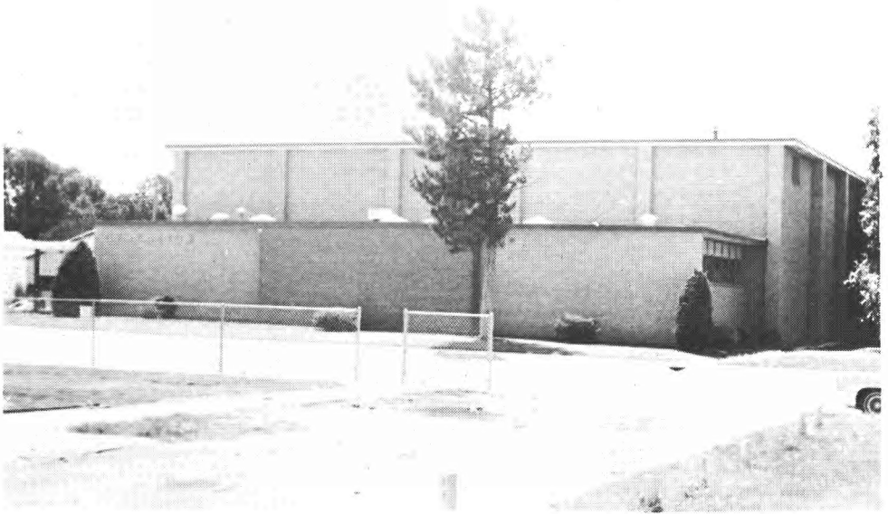
High School Gymnasium
