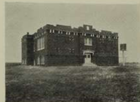
COVERT RURAL HIGH SCHOOL, COVERT, KANSAS.
