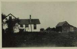
RESIDENCE AND BARN OF JOHN E. BOLAND, ALTON, KANSAS.
