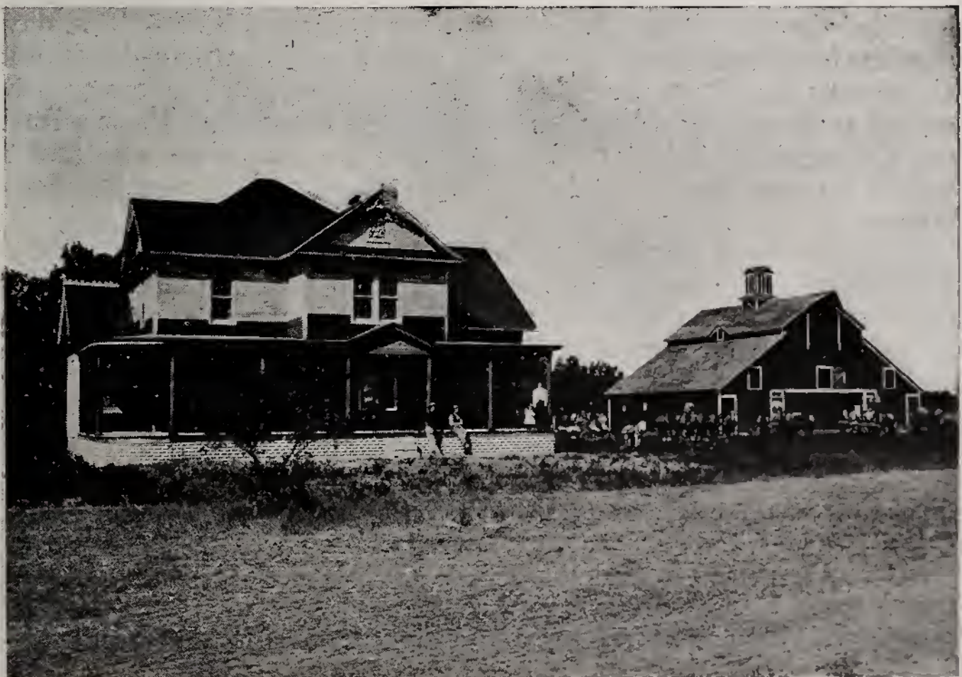
Farm home of Roy Jennings, west of Larned, Kansas. Equipped with steam heat, acetylene light, pressure tank water system and modern throughout.
