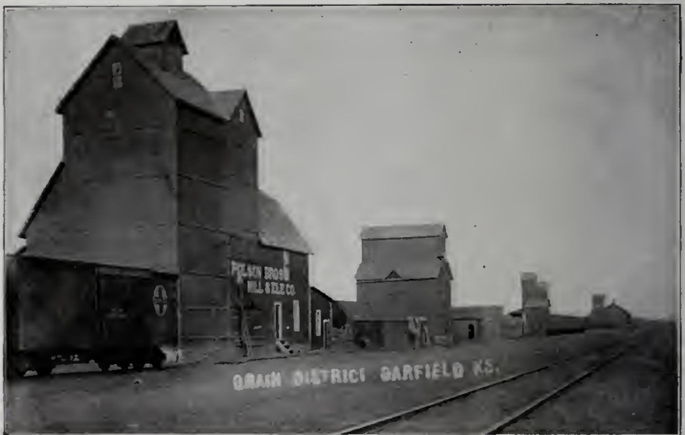
Grain Elevators, Garfield, Kansas
