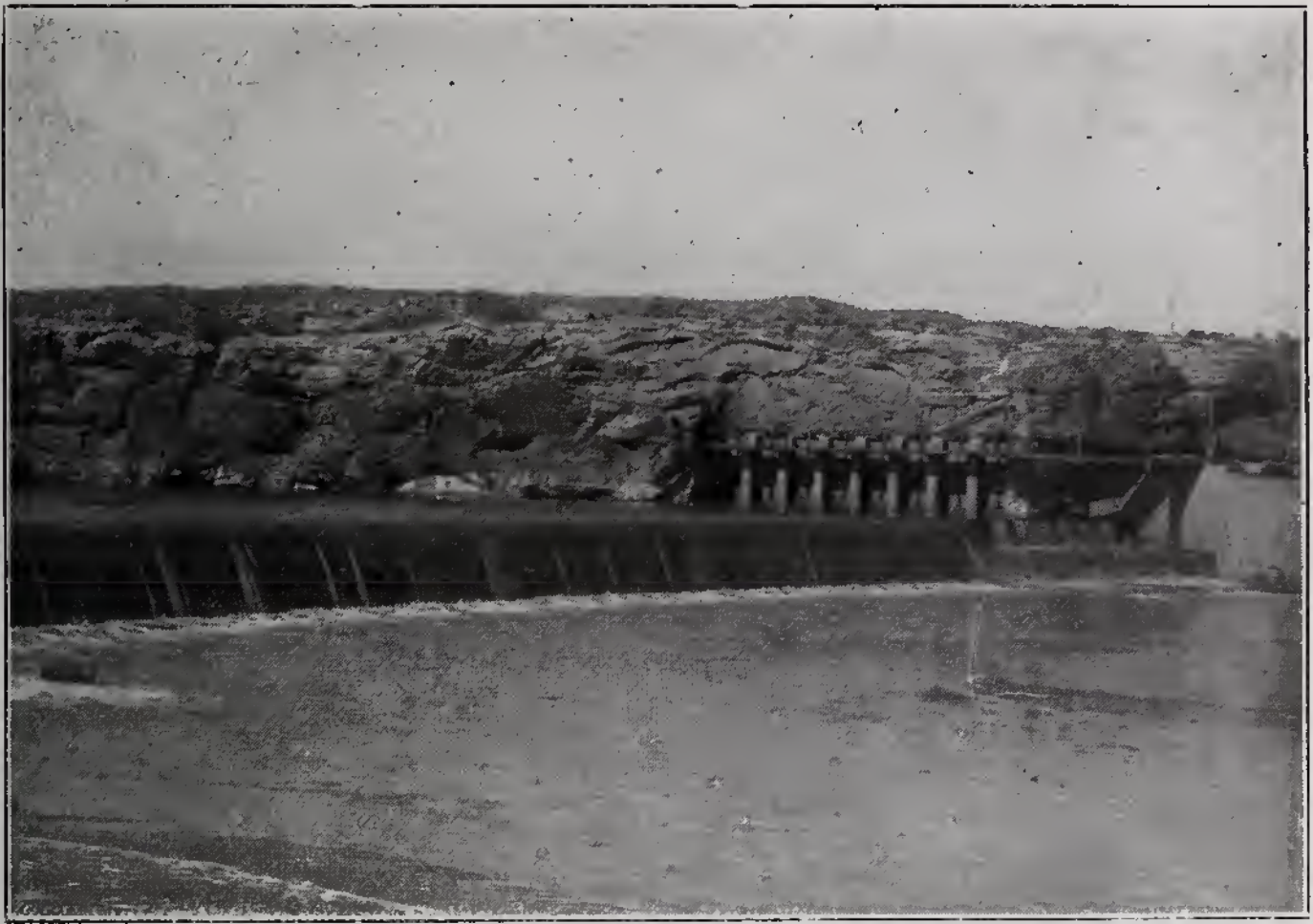
The Amity Canal, Dam and Headgate
