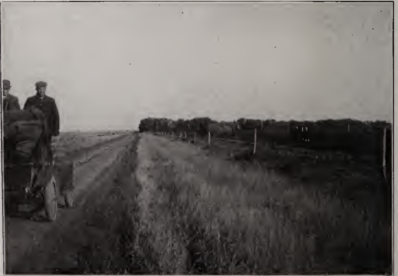
Good Roads on the New Santa Fe Trail
