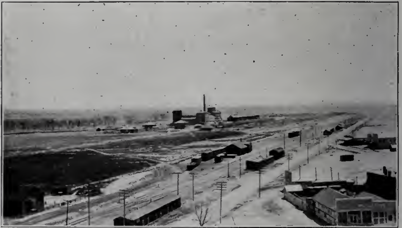
Looking East Toward Sugar Factory at Swink, Colorado, from Water Tank
