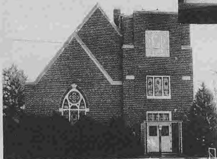
MARCY C. Norris Memorial United Methodist Church in Burdett.
