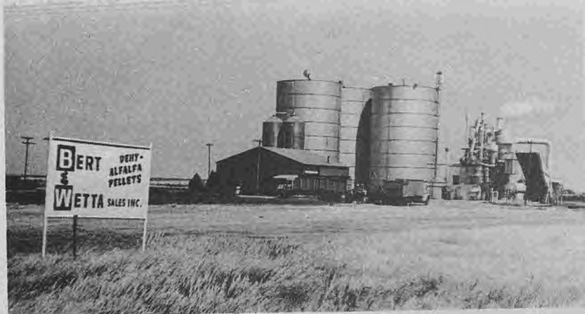
Our 12-year-old facility near Rozel.
