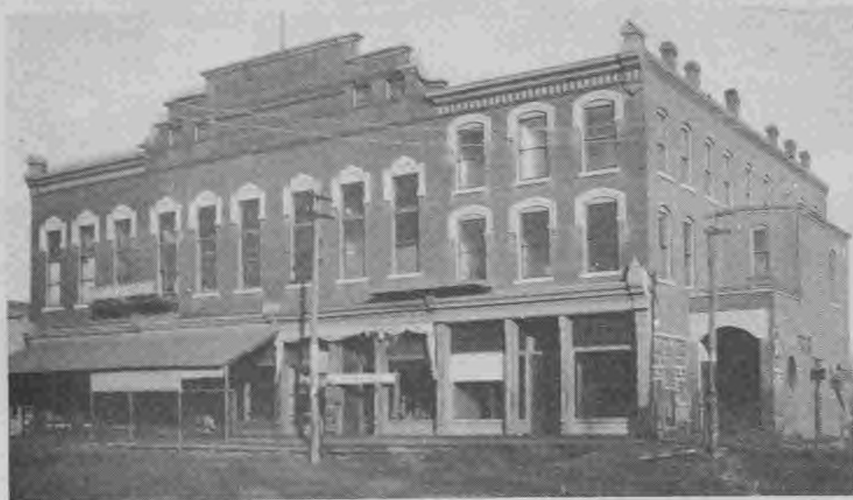
Opera house after completion with crowning cornice work.
