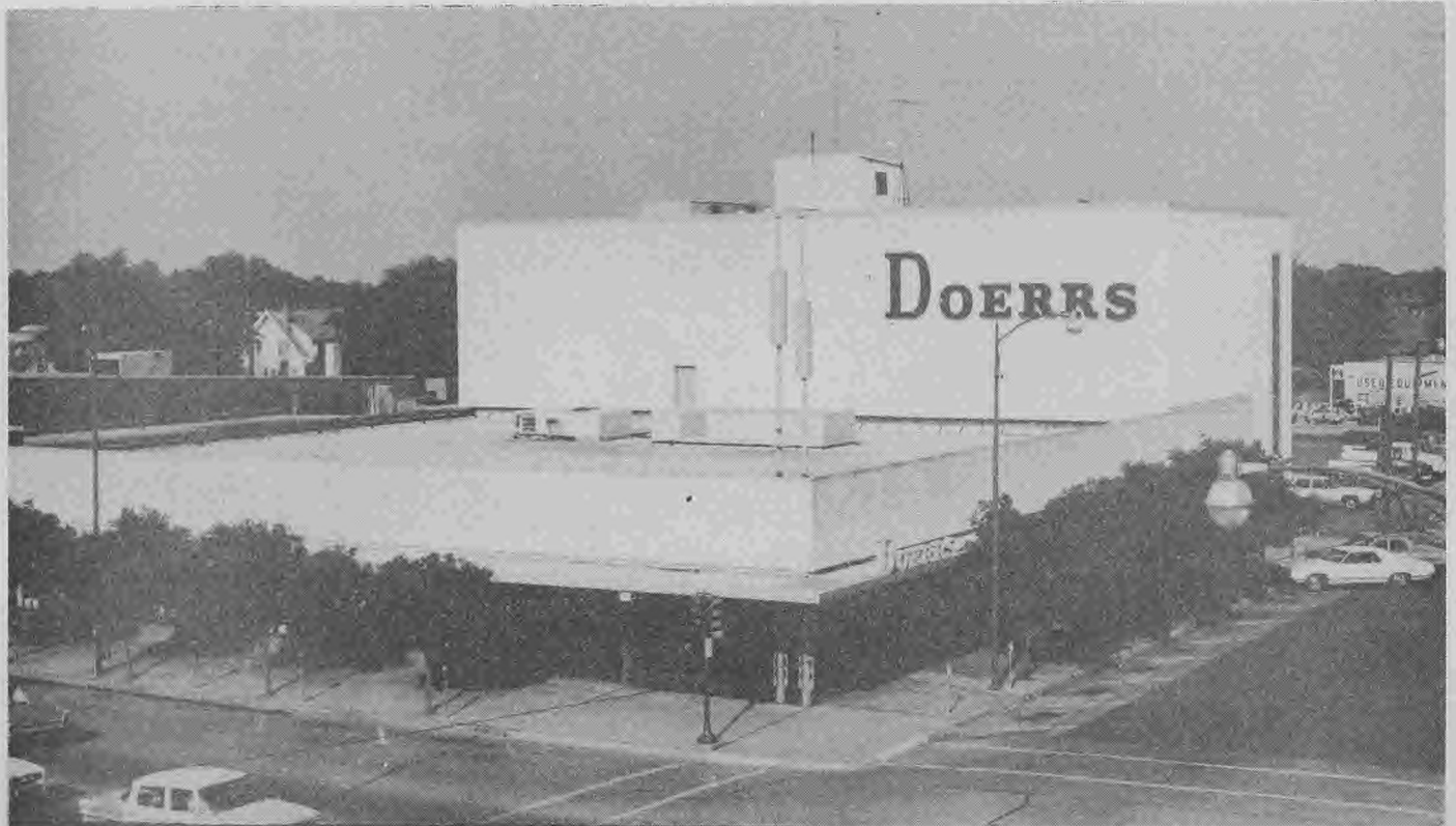
Our building today.
