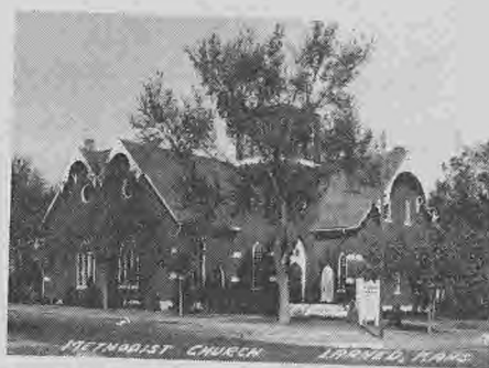
LATER additions covered most of original structure.
