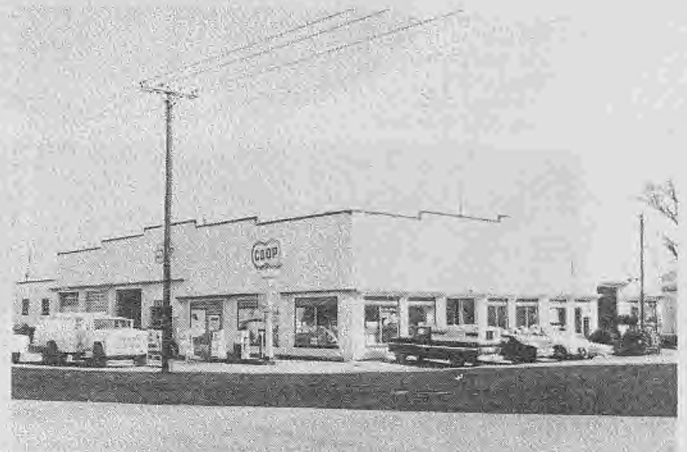
Modern Service Station, Tire & Battery Department
