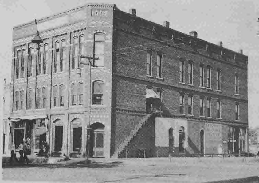
Same building about 1910 with metal cornice removed.
