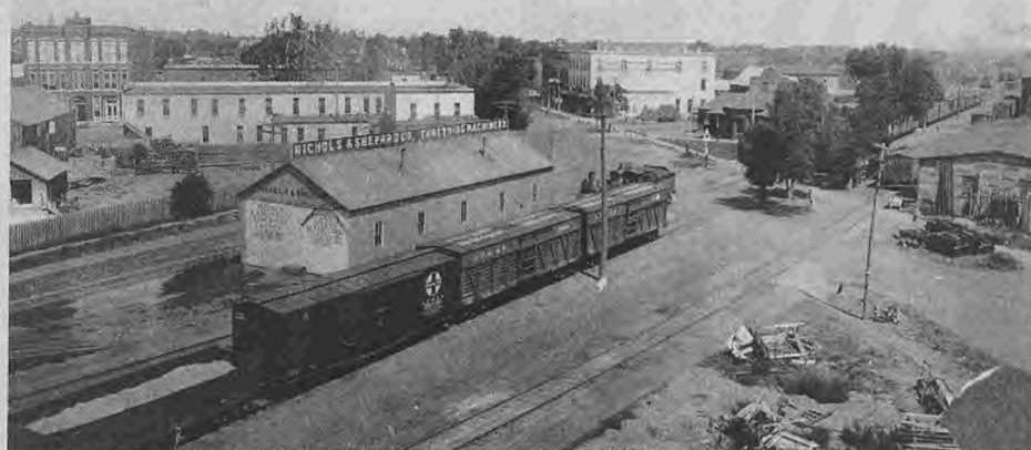
Implement warehouse formerly was located on right-of-way near Broadway.
