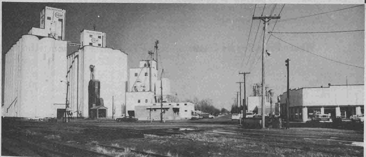
CO-OP FACILITIES expanded to embrace many products and services
