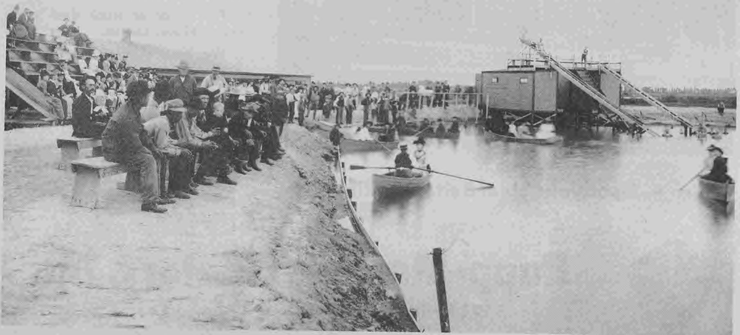
Stands were constructed for use by spectators at salt lake events.
