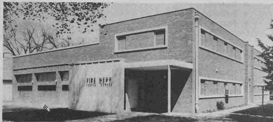
John Schnack Fire Station houses present department and ambulance service.
