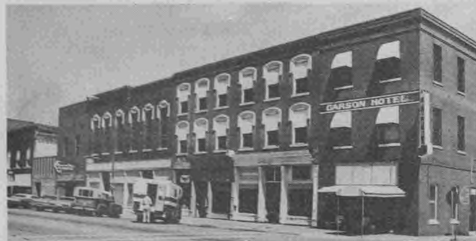
1976 Broadway scene showing remaining opera house structure.
