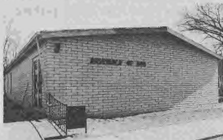
ASSEMBLY OF GOD now meets in this modern structure at Ninth and Topeka Streets.
