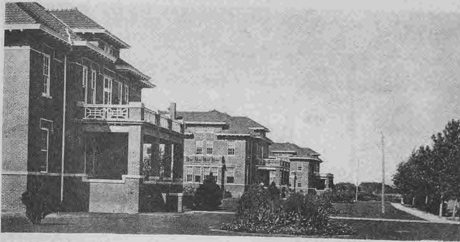
THREE dormitory buildings are shown here soon after completion.
