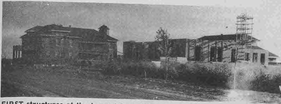
FIRST structures at the Larned State Hospital when it was established was a patients' dormitory and the dining hall seen here under construction.
