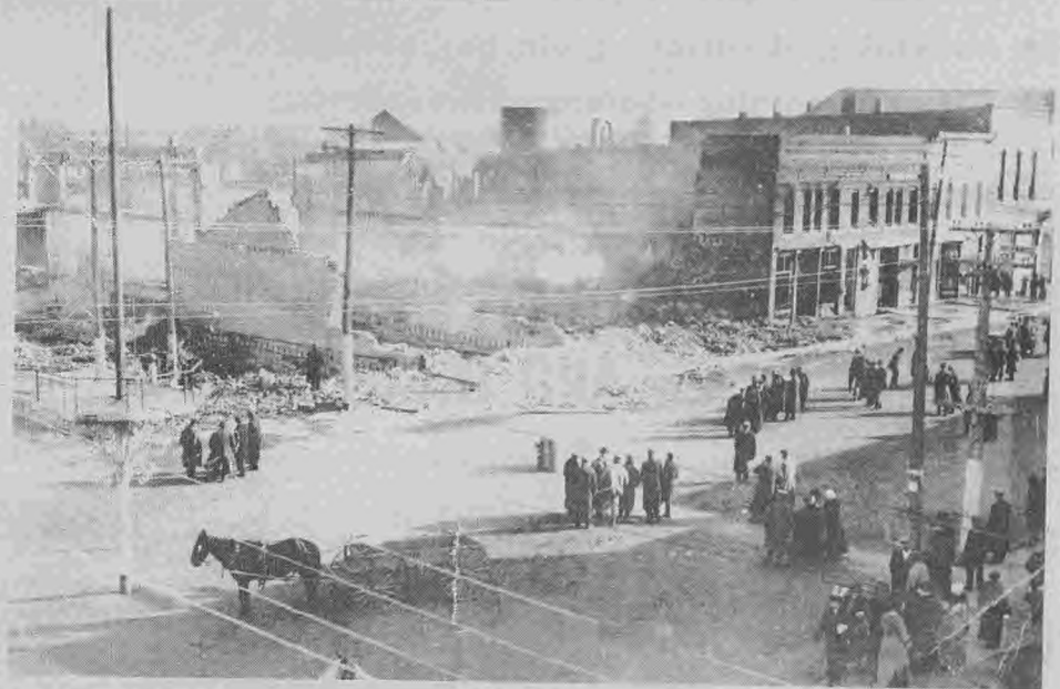
The morning after the January 13 fire.
