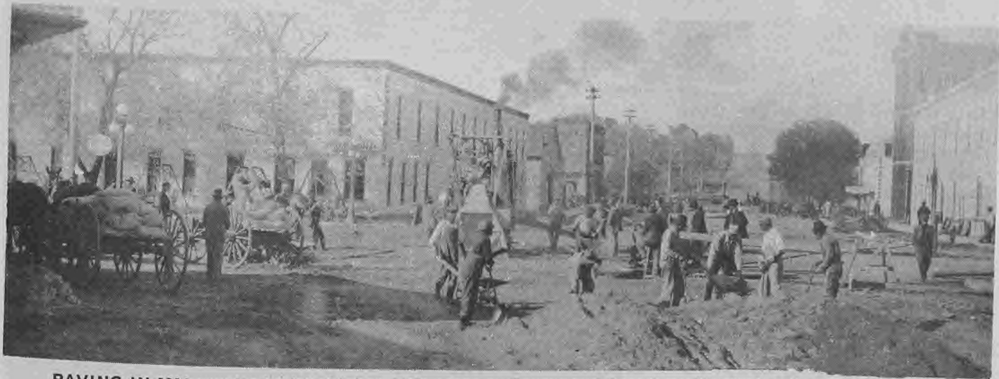
PAVING IN 1916 required a lot of labor. This scene at Fourth and Broadway illustrates the operation.
