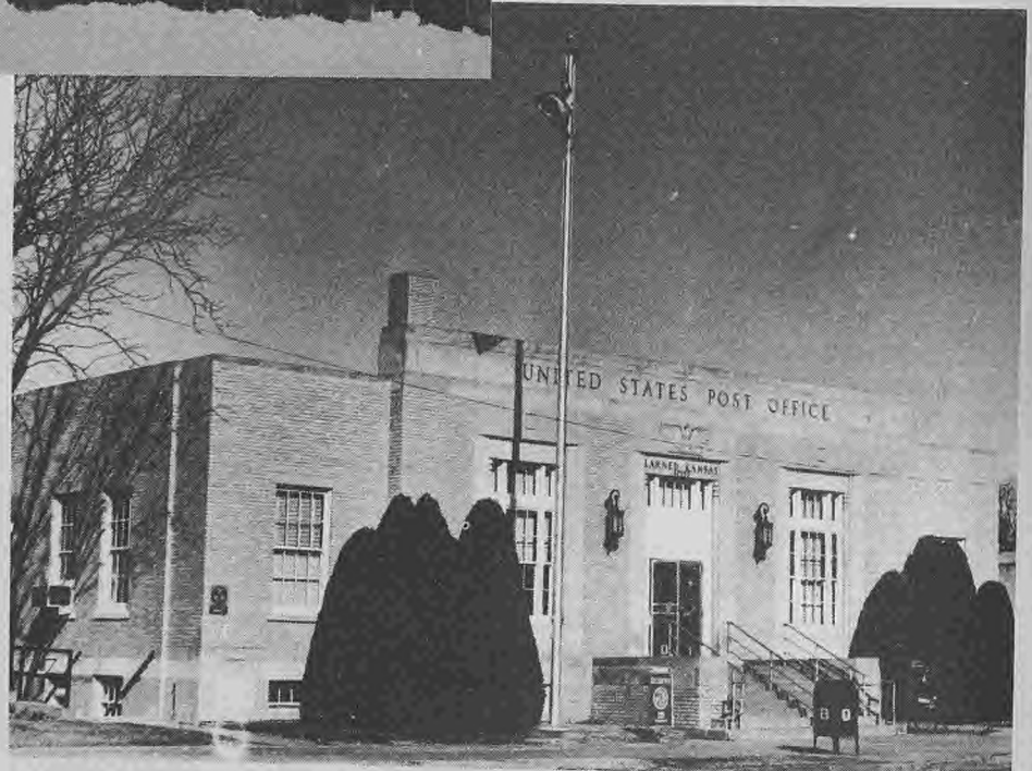
FINAL MOVE came in the 1930s into this government-built structure which continues to house the Post Office at Eighth and Broadway.
