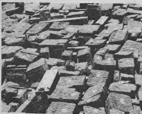
PART of reconstruction and stabilization was a jig saw puzzle.
