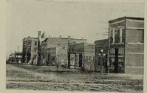
SOUTH SIDE OF SQUARE, LOOKING EAST, PHILLIPSBURG, KANSAS.
