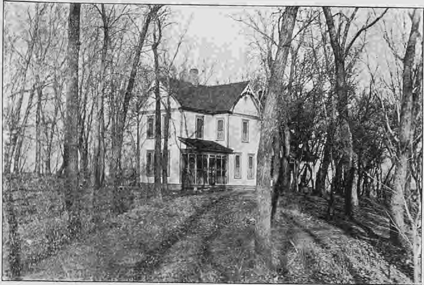
J. C. Bergner & Sons' Ranch House.
