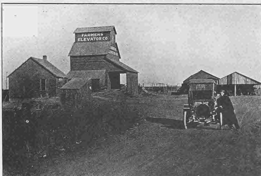
Elevator and Lumber Shed of Farmers' Elevator Co., Cullison, Kansas.
