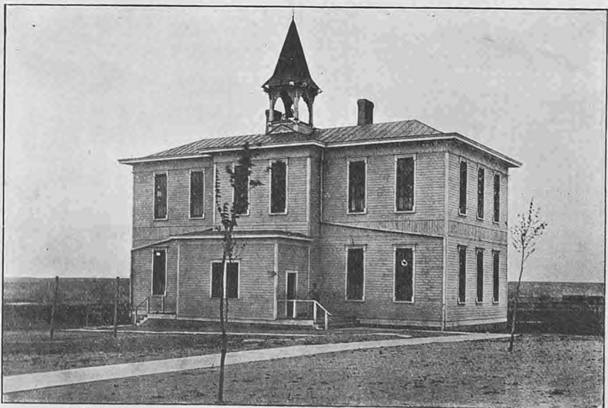
South School Building, Pratt, Kansas.
