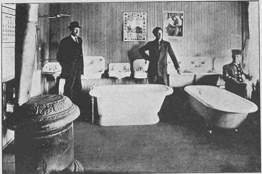
C Office of W. L. McCONNELL PLUMBING AND HEATING CO., Pratt, Kansas. C
