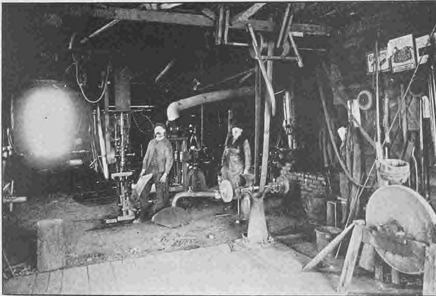
Alex Nickerson's Blacksmith and Wheelwright Shop, Pratt, Kansas.
