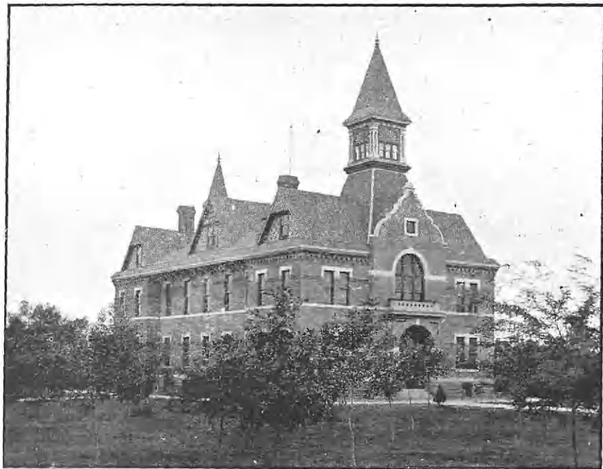
Republic County Court House, Belleville, Kansas.
