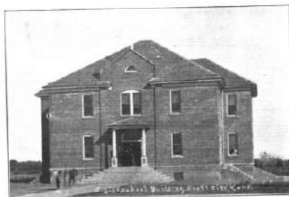
SOUTH SIDE SCHOOL BUILDING, Scott City, Kansas
