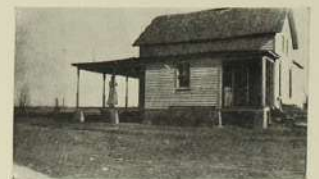
RESIDENCE OF GEO. WRIGHT, KENNINGTON, KANSAS.
