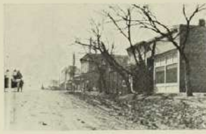
WEST SIDE OF MAIN STREET, LOOKING SOUTH, SMITH CENTER, KANSAS.
