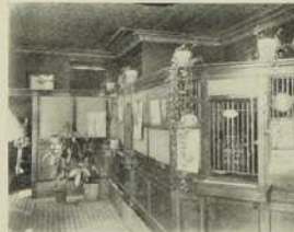
INTERIOR VIEW OF THE FIRST STATE BANK ATHOL, KANSAS.
