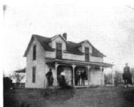
RESIDENCE OF JERRY LONG.
