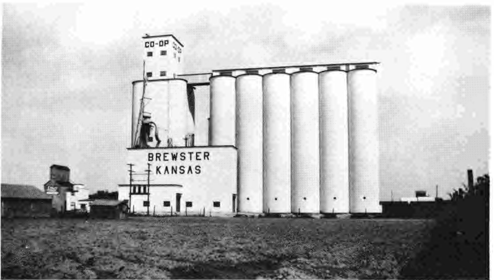
One of the first concrete elevators in Thomas County, 1950.
