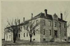
WABAUNSEE COUNTY COURT HOUSE, ALMA, KANSAS.
