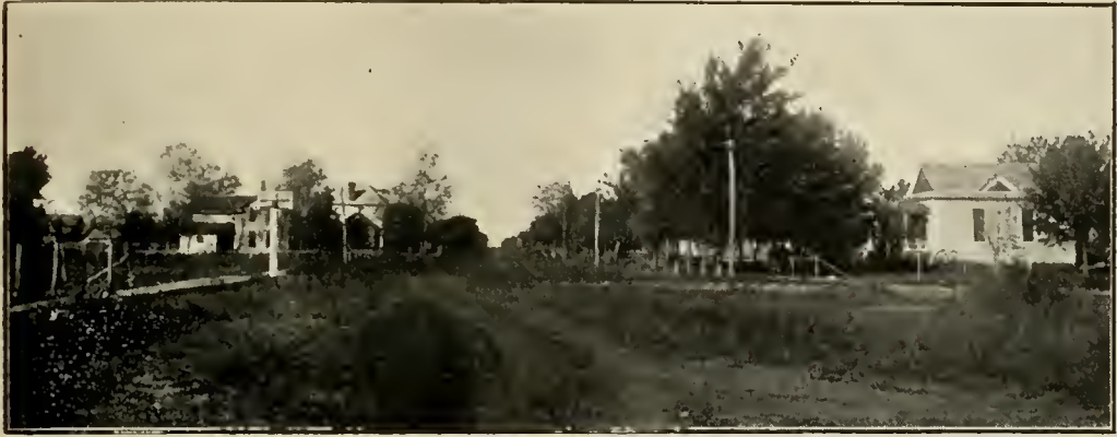
ALMA—LOOKING WEST FROM THE SANTA FE DEPOT.
