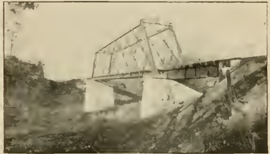
ROCK ISLAND BRIDGE, MAPLE HILL.
