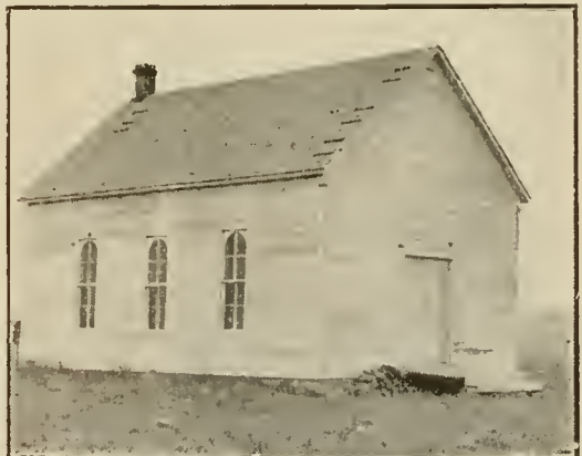
SWEDISH LUTHERAN CHURCH, Mill Creek Township.
