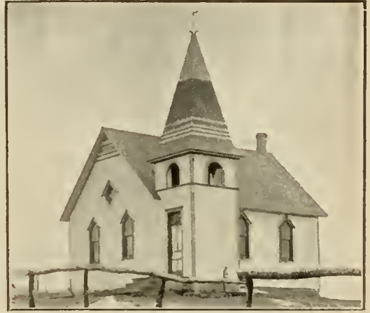
LUTHERAN CHURCH, Kaw Township.
