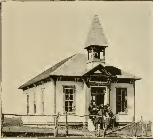
FRAME SCHOOL-HOUSE, Wabaunsee.
