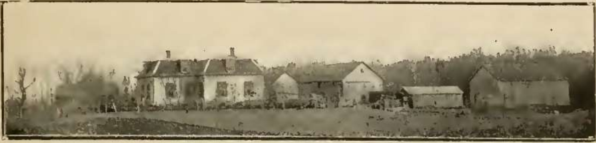
MR. AUGUST ZECKER'S RESIDENCE AND FARM BUILDINGS, near Alma
