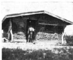
FIRST SOD HOUSE BUILT ON THE RANCH OF THOS. MADIGAN.
