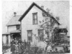
Farm Residence of CARL OESTREICH Linn Township.
