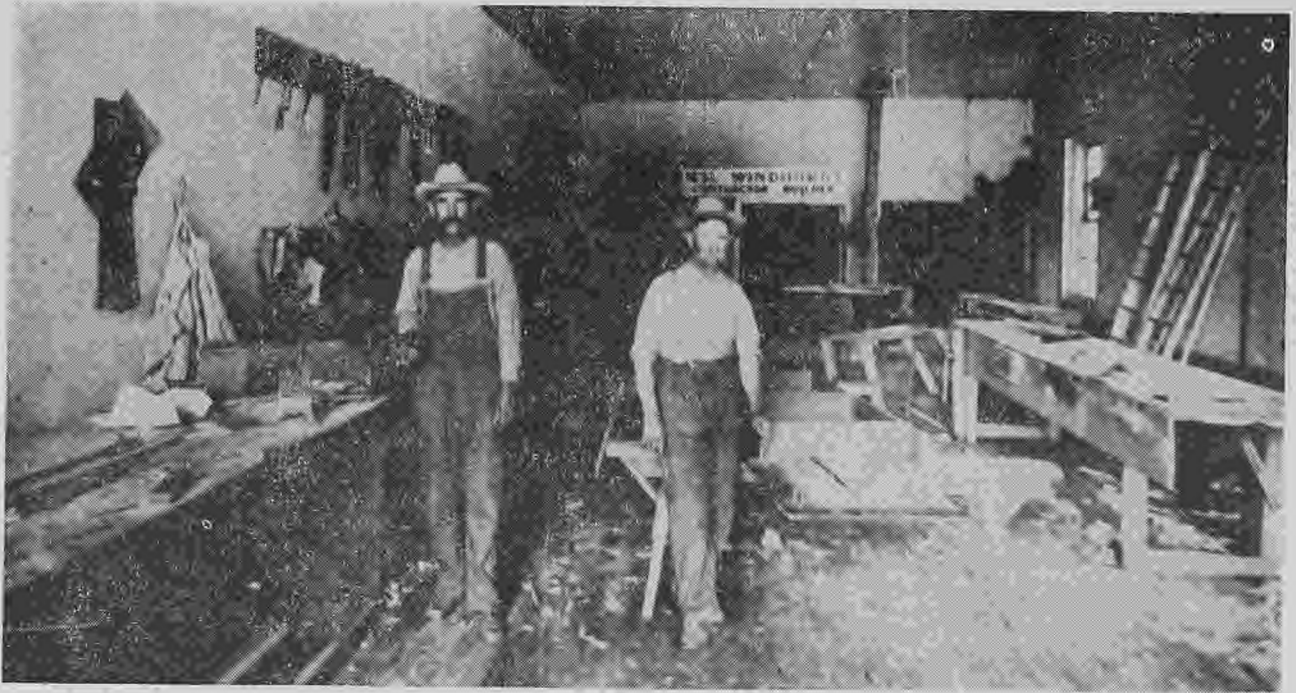
The Windhorst Contracting Shop—At left is Henry Windhorst; right, Jim Arnett
