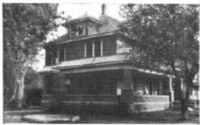
RESIDENCE OF C. A. STAFFORD.
