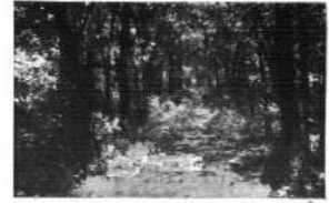
A VIEW ON TOP OF A RAILWAY EMBANKMENT, Built in 1875, 18 to 20 feet high, showing trees covering same. This embankment is soon to be used by the Kansas Railway Co. for an electric line.
