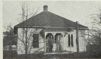
REAR VIEW OF RESIDENCE OF J. A. BRYANT, BETHANY, MO.
