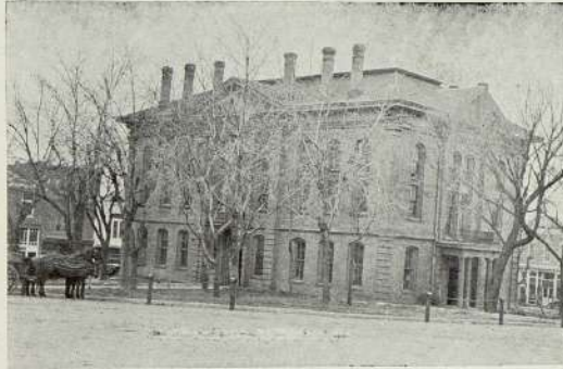
HARRISON COUNTY COURT HOUSE, BETHANY, MO.
