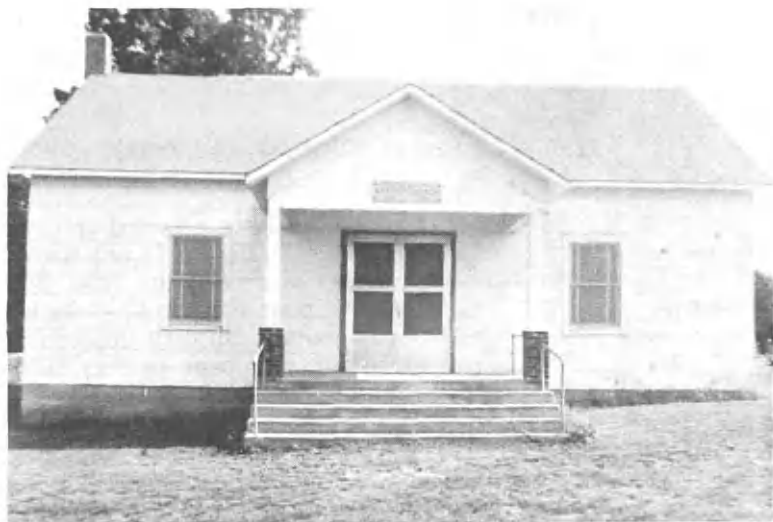
PITTSBURG BAPTIST CHURCH. Organized in 1871, this structure was built in 1956.
