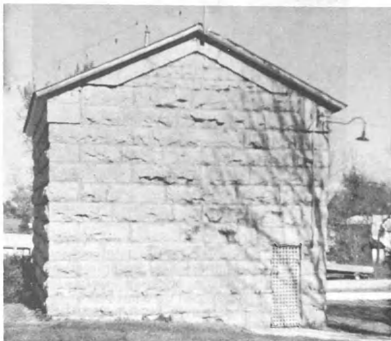
HICKORY COUNTY JAIL BUILT IN 1870
