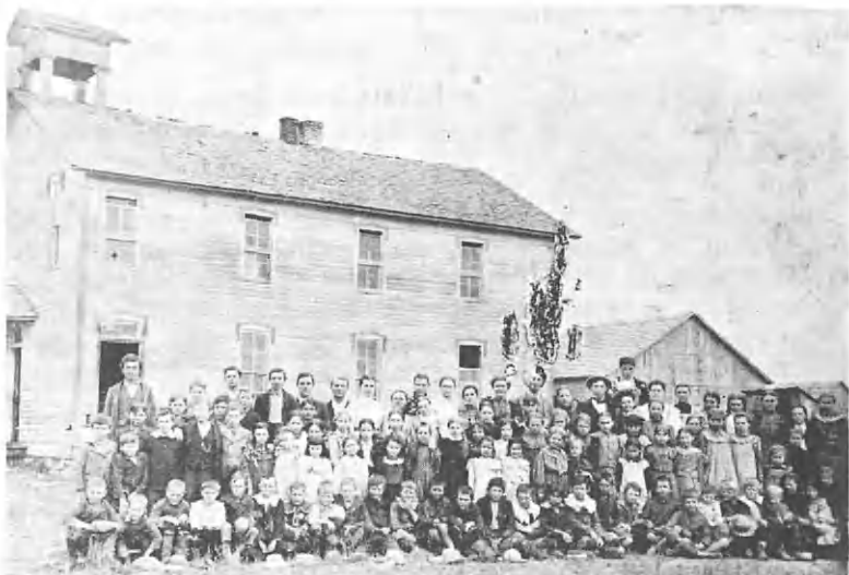
FIRST SCHOOL BUILDING AT CROSS TIMBERS
