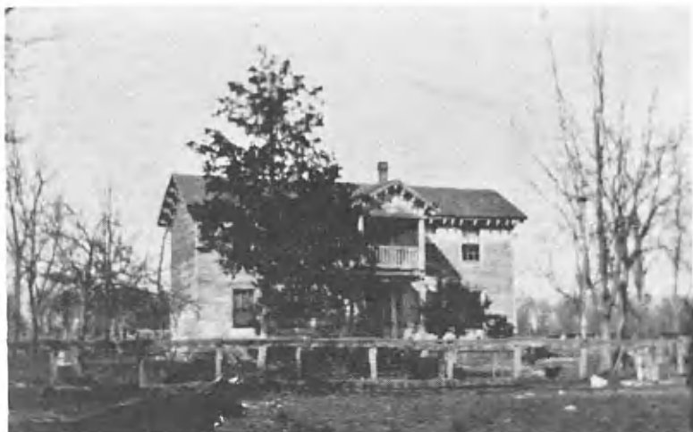
JOHN W. QUIGG RESIDENCE BUILT IN 1860's North of Wheatland.
