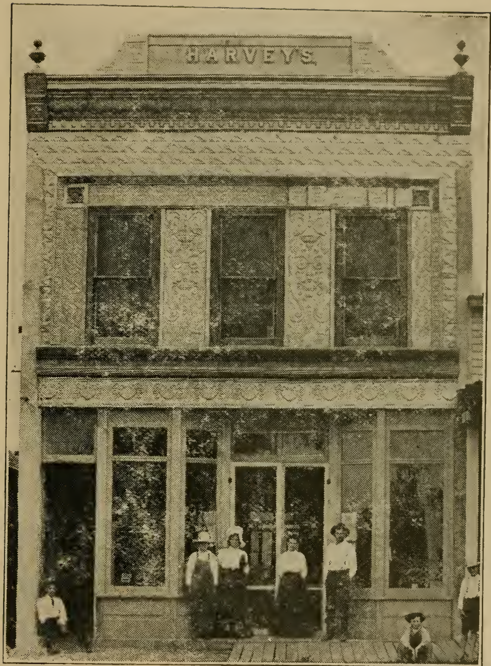
J. E. HARVEY'S BUSINESS BUILDING, Cross Timbers, Missouri.
