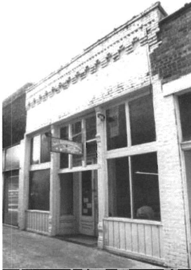
Figure Sixteen. L. D. Harlin Building, 2 Court Square Photo by Becky Snider
