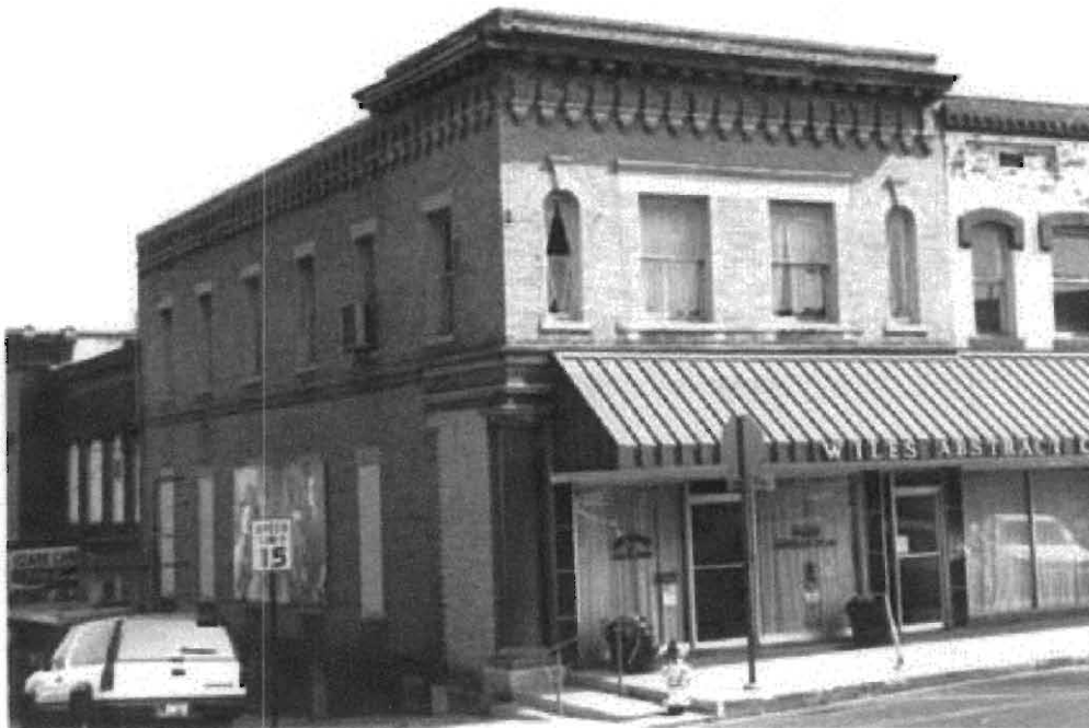
Figure Eight. G. H. Carter/Howell County Bank Building, 20 Court Square Photo taken by Becky Snider, 2000.
