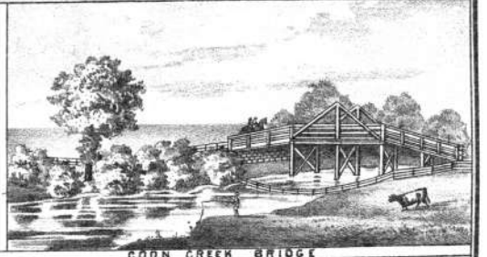
COON CREEK BRIDGE
