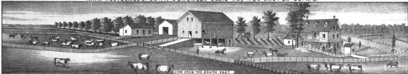
VIEW FROM THE SOUTH EAST
