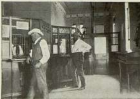
INTERIOR VIEW, CLARK EXCHANGE BANK CLARK, MO.
