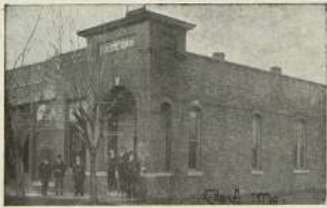
EXTERIOR VIEW, CLARK EXCHANGE BANK CLARK, MO.
