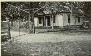
RESIDENCE OF G. R. DAVIS, BLACKBURN, MO.
