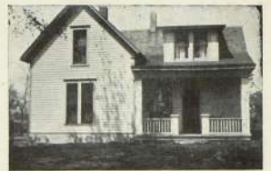
RESIDENCE OF TABLER BROS., NORTON, MO.
