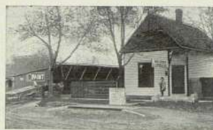
LUMBER YARD OWNED BY W. O. LIESER, BLACKBURN, MO.
